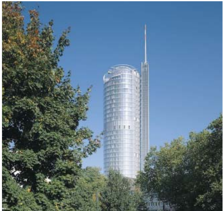
Fig 2 A speech-making double-skin facade, the first one in Germany, is the 127 m high RWE tower in Essen. The architects provided this cylindrical high rise building, diameter 32 m, with 7000 m 2 of double-skin facade. The total facade surface area comes to 17.000 m 2 . Photo: Gartner
