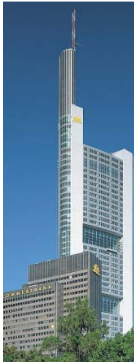
Fig 13 The 1991 prize-winning design for the Commerzbank in Frankfurt am Main in Germany reflects the client's concern to produce an ecological, low-energy building Photo : Gartner
