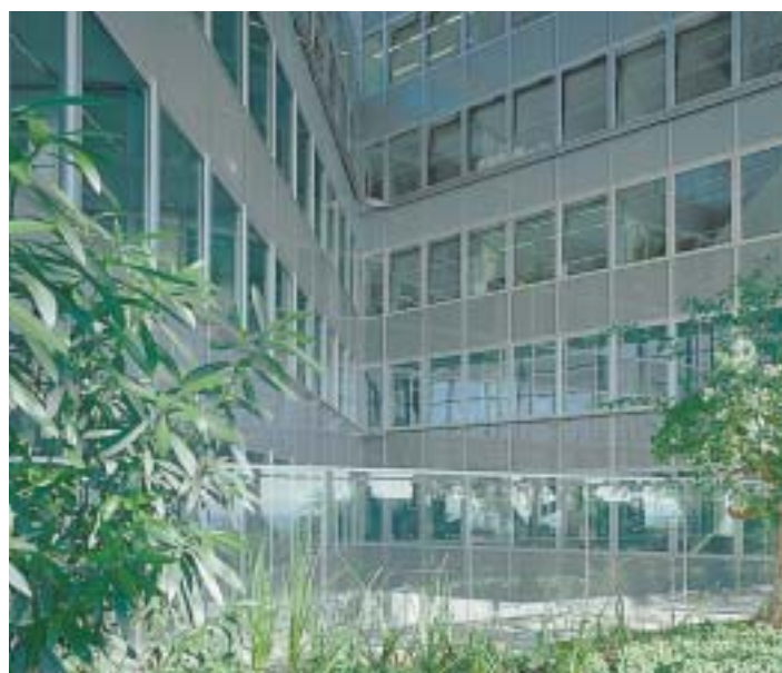
Fig 14 For this project two variations on the principle of the "buffer zone" for natural ventilation of the offices were used : as a double skin facade and as a winter garden Photo : Gartner
