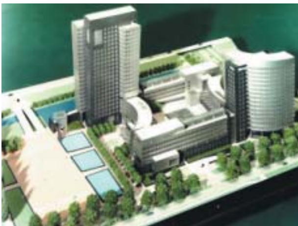
Fig 7 The head office of ABN-AMRO in Amsterdam is provided with 24200 m 2 of climate facade. Photo: Capital Press
