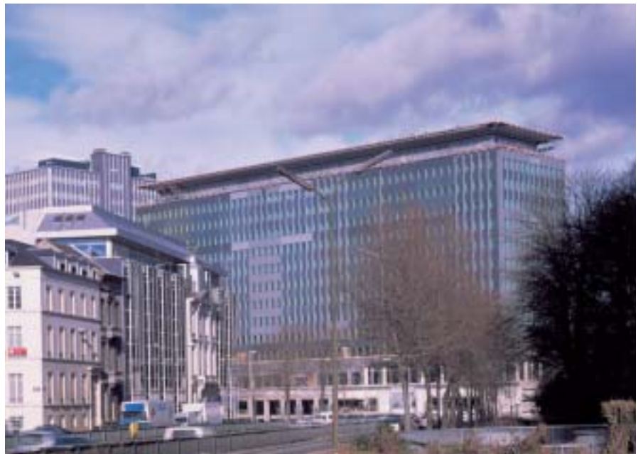
Fig 1 Dexia Bank in Brussels. The Climate Facade technology utilised for this refurbishment of 34.000 m 2 of office accommodation comprised a factory prefabricated curtain wall type facade, consisting of a double outer and single inner glazing with solar protection in between. The overall thickness of the facade was about 180 mm with easy access to the inner glazing for cleaning purposes.
