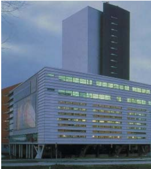
Fig 11 National Nature-Historical Museum 'Naturalis', Leiden An exceptional design of a climate facade is used in the depository tower. In order to reduce the influence of the outdoor climate to an absolute minimum there is no glass opening whatsoever in the facade and the air cavity is ventilated by an air-conditioned system. Photo: VROM
