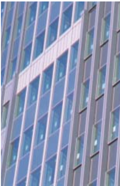
Fig 1 Dexia Bank in Brussels. The Climate Facade technology utilised for this refurbishment of 34.000 m 2 of office accommodation comprised a factory prefabricated curtain wall type facade, consisting of a double outer and single inner glazing with solar protection in between. The overall thickness of the facade was about 180 mm with easy access to the inner glazing for cleaning purposes.
